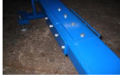
Figure 2. Fish plate joining section
